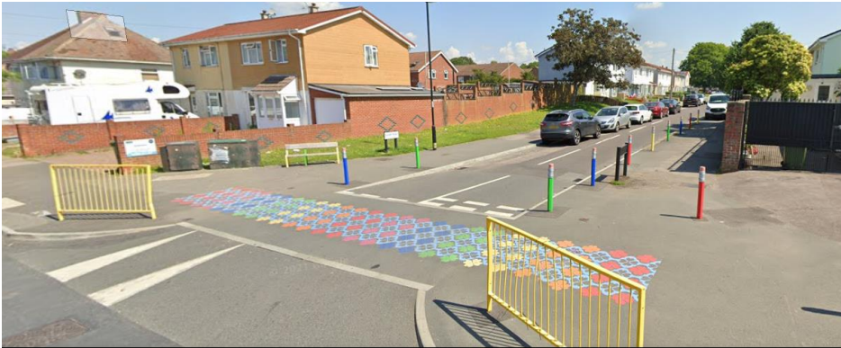
Further safety measures and area improvements in 2021
